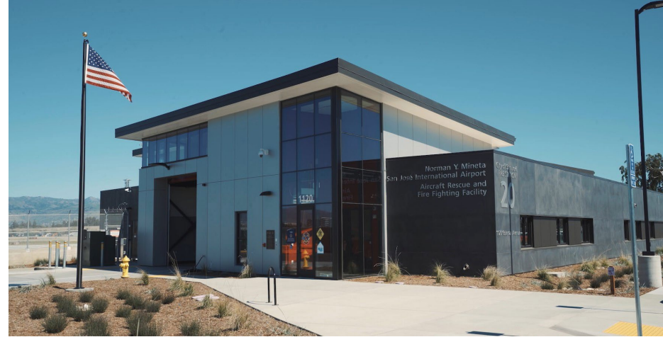
ARFF Station 20 from Coleman Ave.
