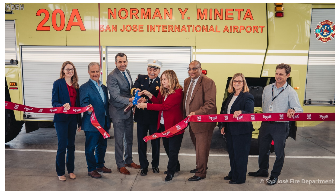
Completed New ARFF facility which was designed and constructed to LEED Silver standards. Some of its sustainable attributes include EV charging stations, a cool roof, uses drought-tolerant xeriscaping, and is net zero carbon and net zero ready.
