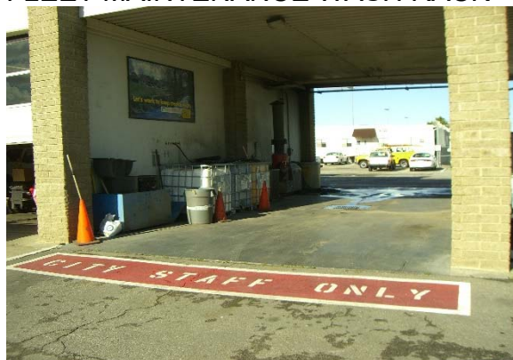
FLEET MAINTENANCE WASH RACK
