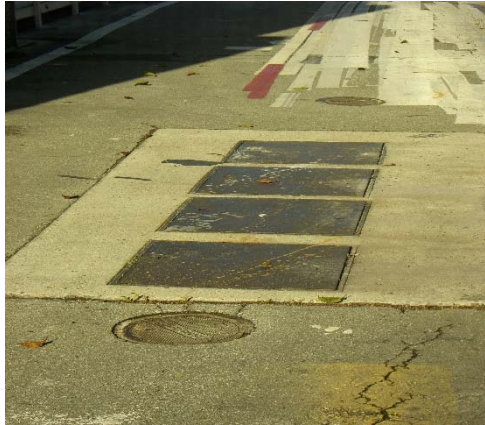
PAINT SHOP CLARIFIERS
