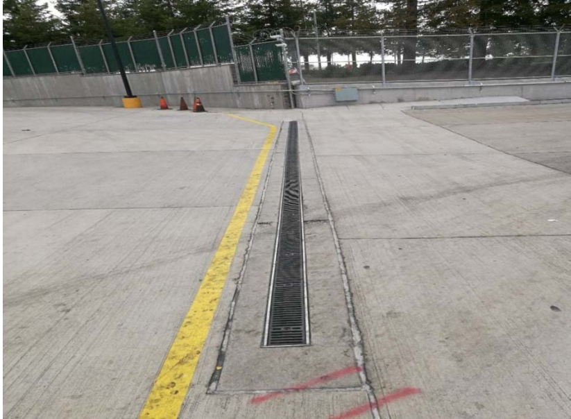
TRENCH DRAIN AT NORTHEAST PARCEL STORAGE AREA
