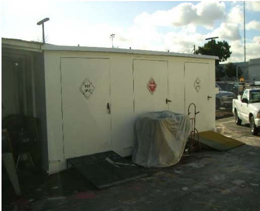
PAINT SHOP STORAGE
