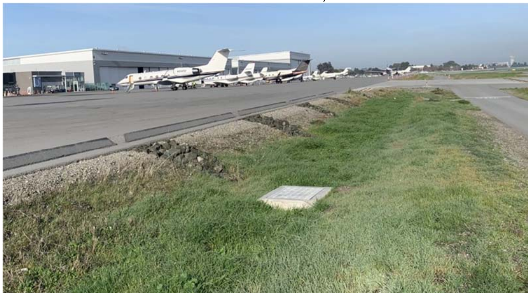
BIORETENTION CELL AT SIGNATURE, FACING NORTH-WEST
