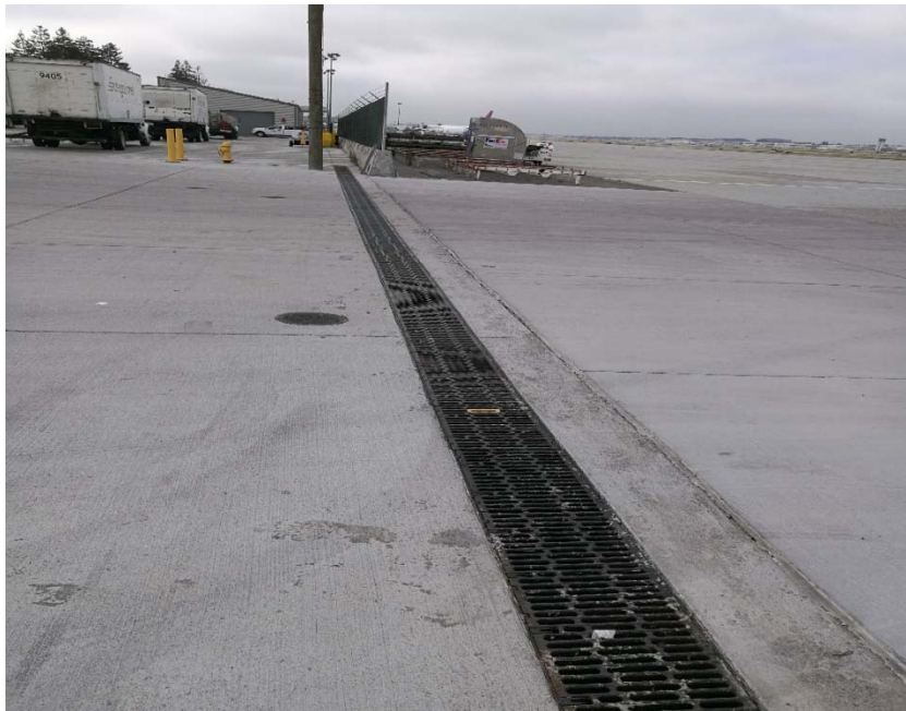
TRENCH DRAIN AT NORTHEAST PARCEL STORAGE AREA
